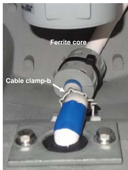
14) Clamp the cable by the cable clamp-b.
