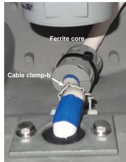
14) Clamp the cable by the cable clamp-b.
