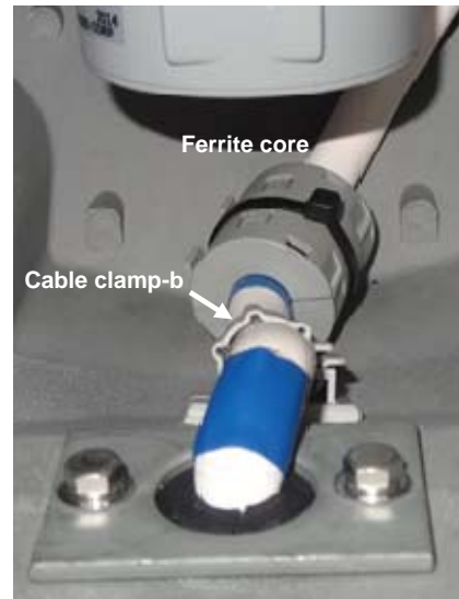
14) Clamp the cable by the cable clamp-b.
