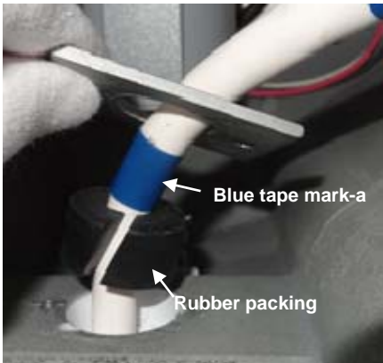
9) Attach rubber packing to the blue tape Mark-a.
