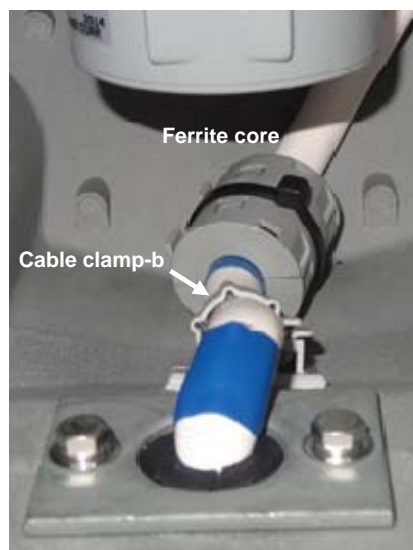
14) Clamp the cable by the cable clamp-b.
